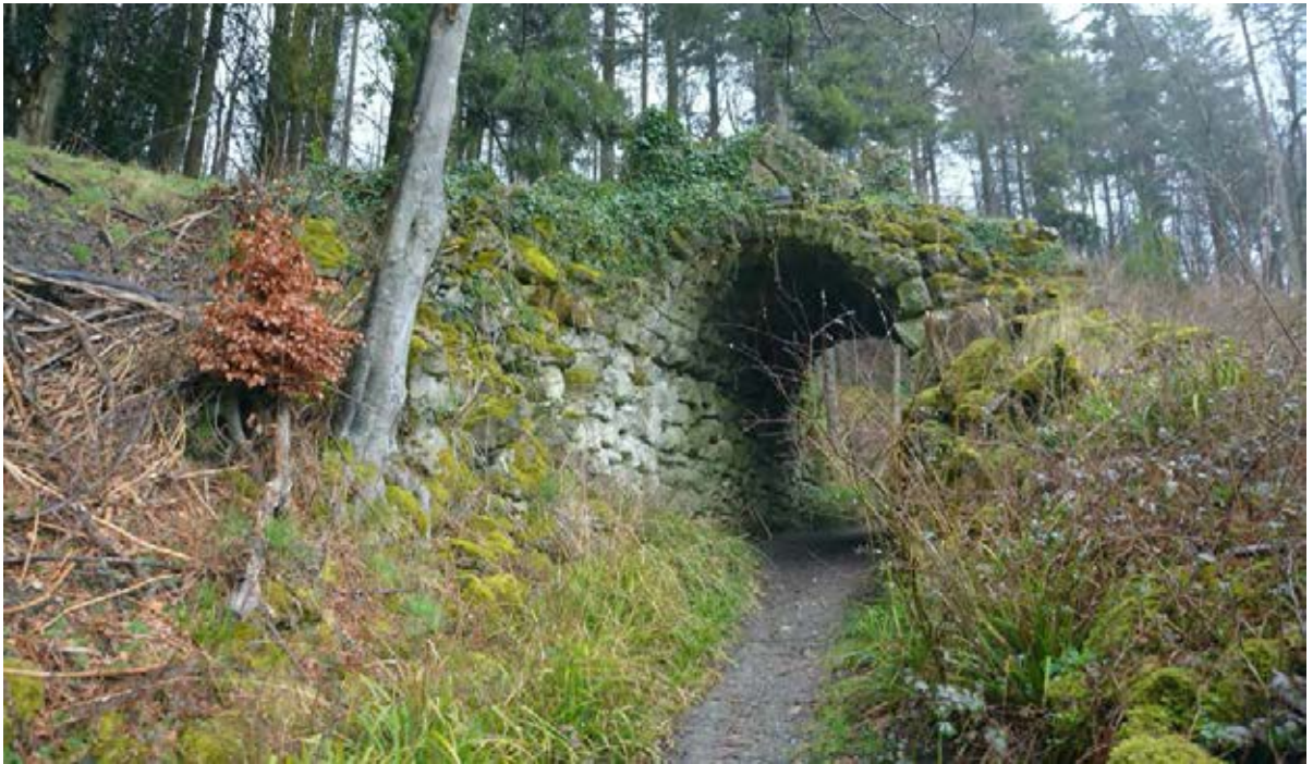
The Rock Arch viewed from the west.
